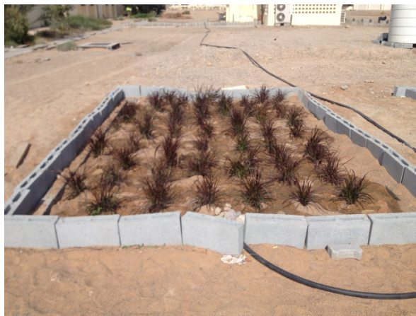
FIGURE 3. The constructed field scale vegetative bioretention systems
